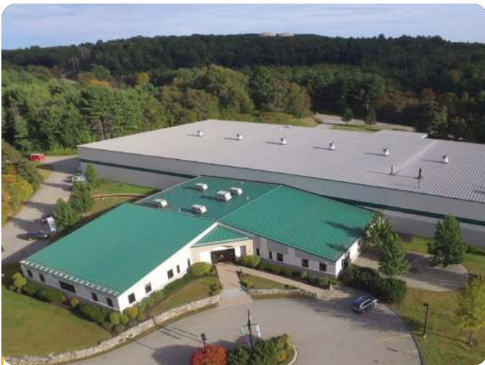
Modula Headquarters and Plant – Lewiston, Maine
